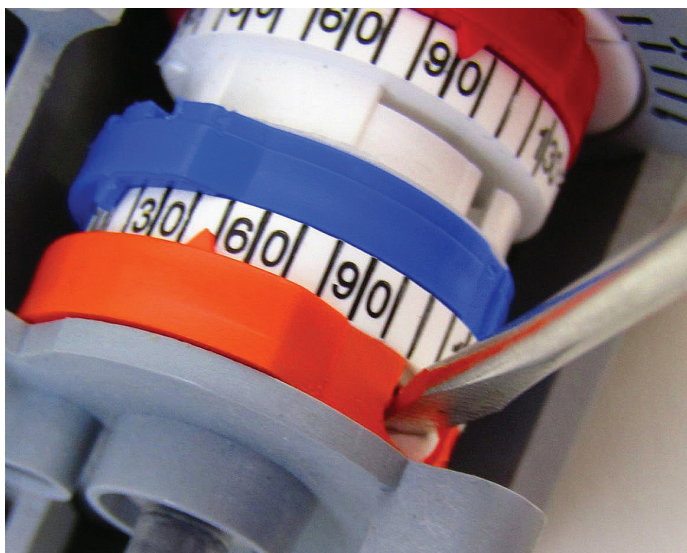
Setting Transition (Orange Cam) Transition cam is set with a screwdriver. Transition should be set half way between High Fire and Low Fire to start. Adjust if necessary.
